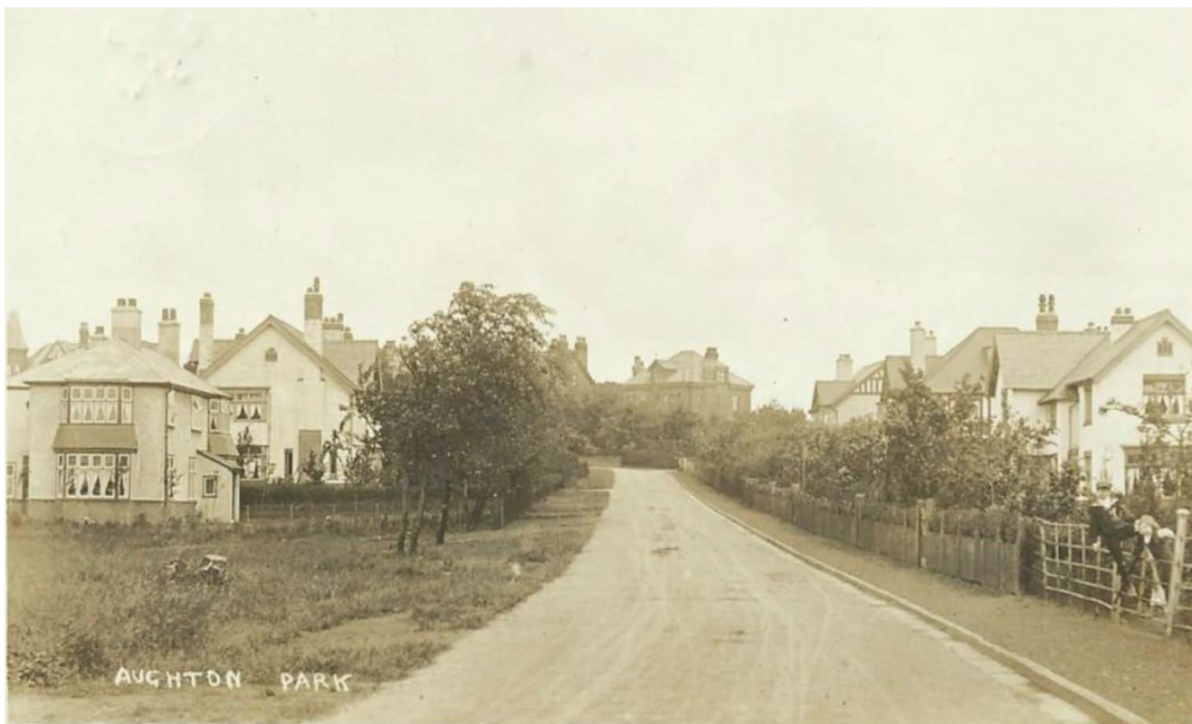
This early 20 th century photograph shows some of the newly constructed phase 2 properties alongside the late Victorian development visible at the head of Granville Park. 7 Granville Park lies on the left of the picture in the foreground, while no.6 is in the right foreground. The vacant plot to the south (later to be occupied by no.5) is also clearly visible.
